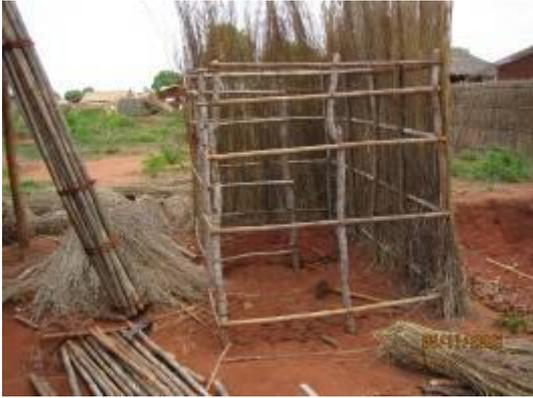
Fig 5: Latrine superstructure under construction
