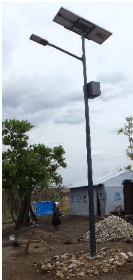
Photograph 1. An installed lamppost
