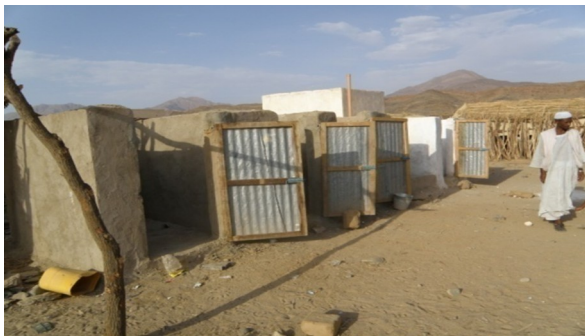
Photo: Public latrines constructed by the community in Halhal village
