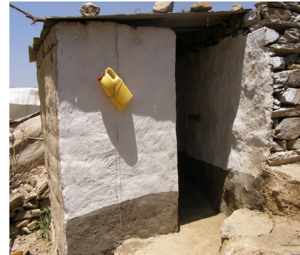
Photo: Locally designed and built Household latrine with hand washing facility
