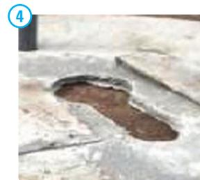
4 The drop-hole is a keyhole shape with slope inwards
