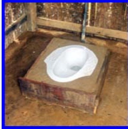
One of the fanciest pour-flush toilets constructed (including solar lighting)
