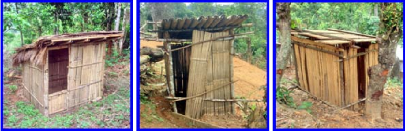
Dry pit latrines constructed after CLTS triggering
