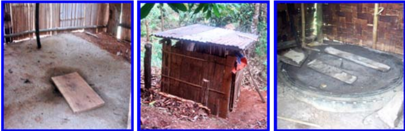
Some properly constructed dry pit latrines
