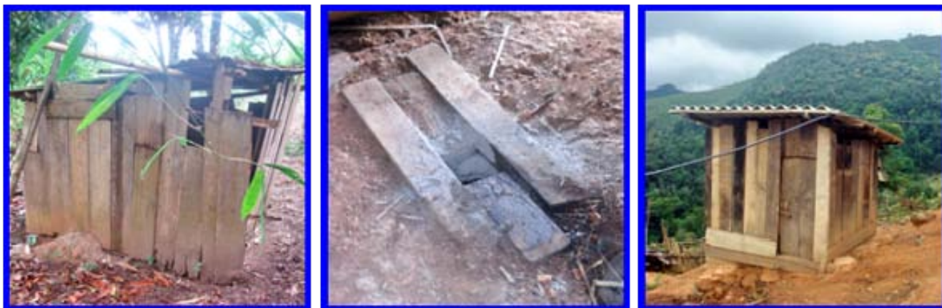
Latrines constructed prior to CLTS triggering
