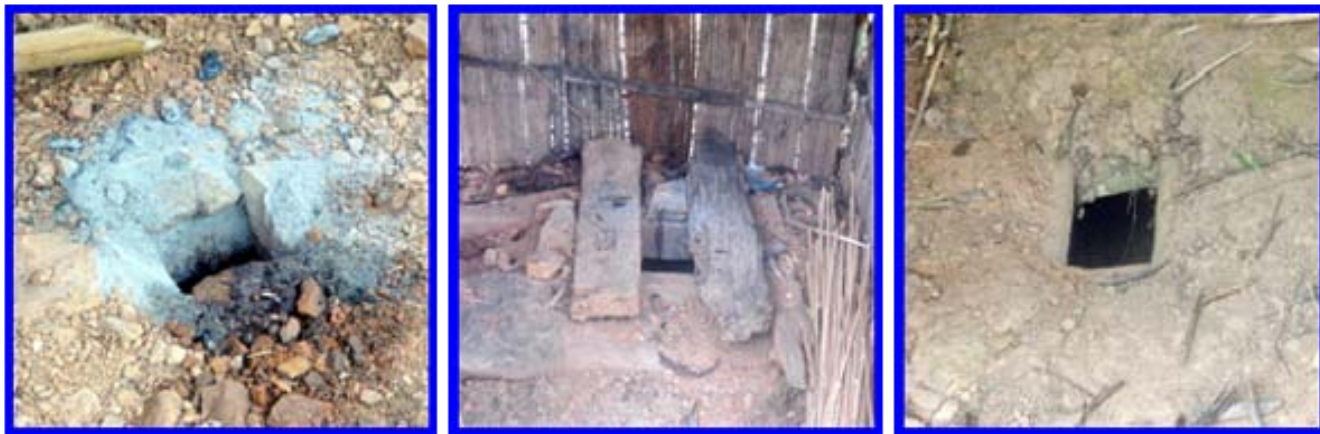
Conditions of some of the dry pit latrines
