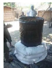
Photograph 3: Wooden frame (nkhokwe) is wrapped in plastic and reinforced with sand-bags
