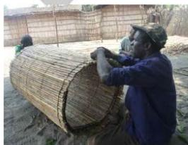
Photograph 2: Wooden frame (nkhokwe) is constructed using local reeds woven with rubber threads taken from tyres
