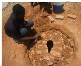
Photograph 1: Top view of prototype of corbelled design
