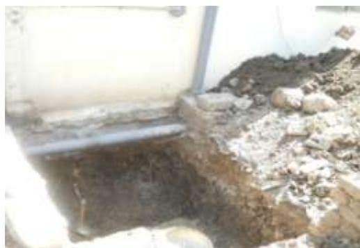
In Amba Nagar locality, many houses have been built under BSUP. The houses have toilets but the use of these toilets had not started as people were waiting for the completion of sewer lines and connection of the toilets to the same. During triggering people realized that they could easily end OD by just making a leach pit outside their houses and connecting it to the toilet till the sewer line gets completed. Some of them were innovative in cutting costs of leach pit by using
