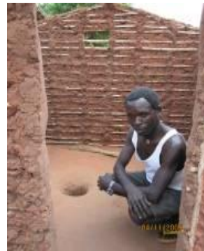
Fig 2: Traditional latrine platform – finished
