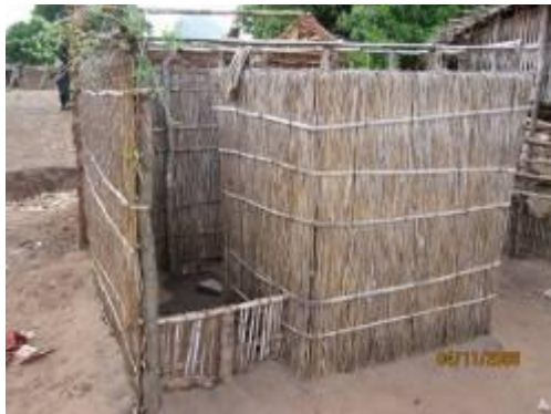
Fig 7: Traditional latrine superstructure
