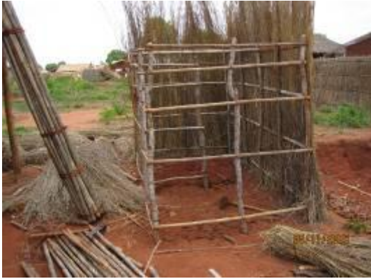
Fig 5: Latrine superstructure under construction
